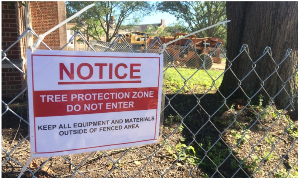
Fig. 5 Signage to be placed on all protective fencing
